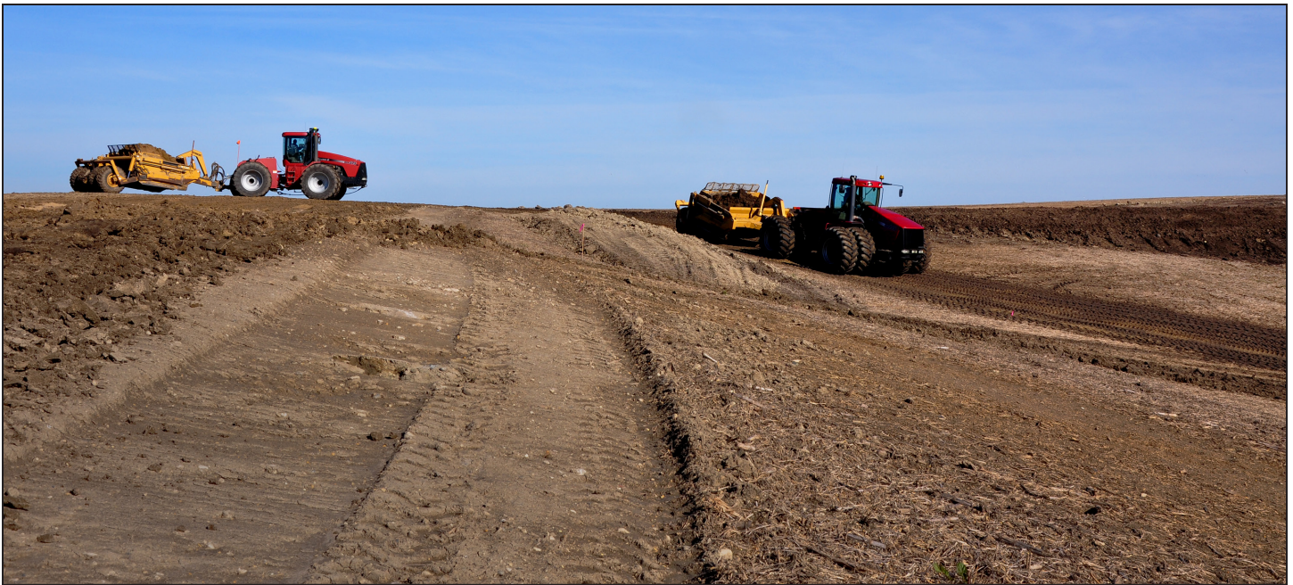
Outlet Creek cuts through Todd (right) and Tom Johnshoy’s field between lakes Minnewaska and Emily. An Erickson Excavating crew shaved clay off a hilltop to construct a series of water and sediment control basins. The structures are part of a Pope SWCD project, which uses a Clean Water Fund grant in an ongoing effort to clean up Lake Emily.
